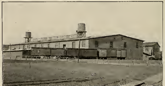
PART OF PRESENT PLANT, WEST END.
